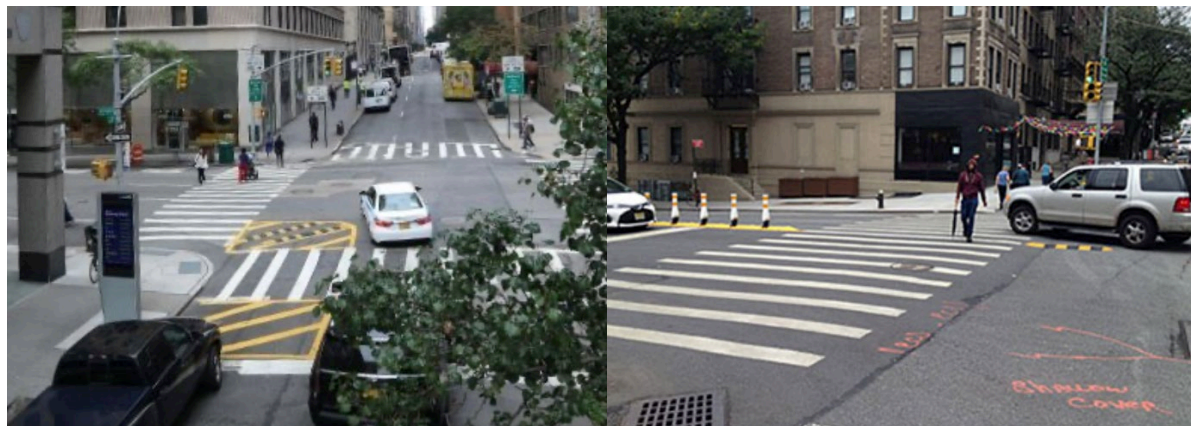
Figure 7 Slow Turn Wedge (left) and Basic Hardened Centerline (right) (Source: NYC DOT, 2024)
