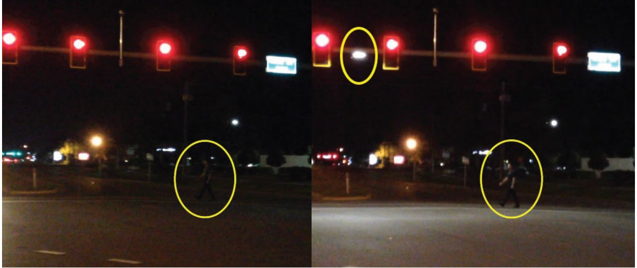
Figure 12 Before (left) and after (right) LED installation for pedestrians dressed in dark clothing (Source: Jeffrey Trombly and Associates, 2019)
