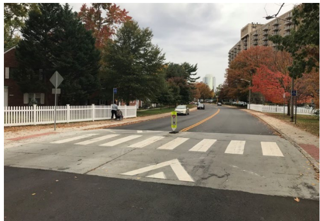
Figure 19 Raised pedestrian crossing (PEDBIKESAFE, 2023)
