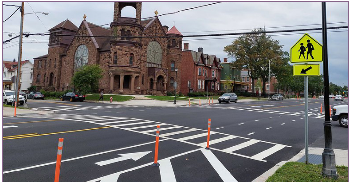
Figure 2. An intersection with pedestrian visibility enhancements and painted bike lanes. ( NJDOT Bicycle and Pedestrian Resource Center )
