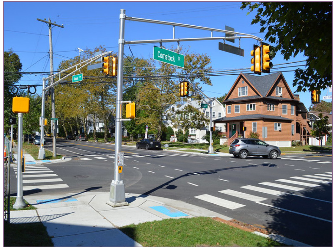
Figure 21. Accessible pedestrian signals can better communicate pedestrians' right of way by combining visual, auditory, and vibrotactile cues that work in concert to convey information about how and when to cross the street. (NJDOT Bicycle and Pedestrian Resource Center)
