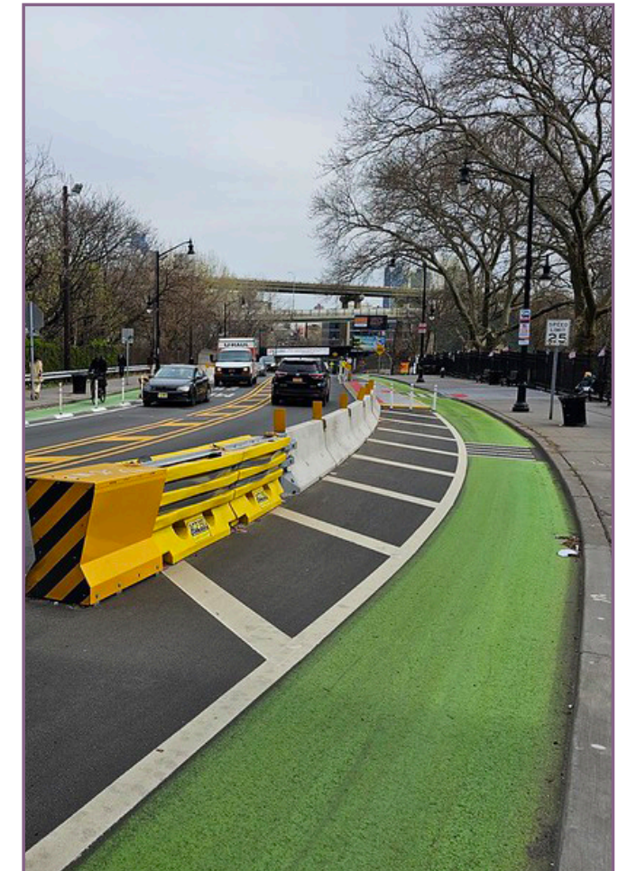
Figure 28. Neurodivergent individuals may benefit from the installation of more protected bicycle lanes and separated bicycle paths that are wide enough to accommodate a variety of device types, such as tricycles. ( NJDOT Bicycle and Pedestrian Resource Center )
