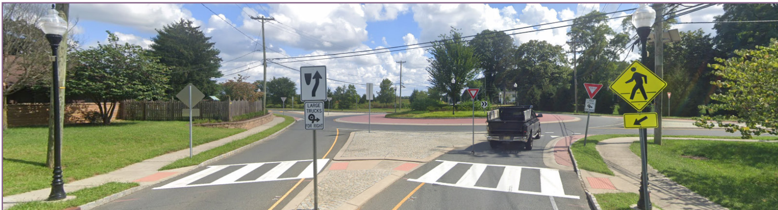
Figure 26. Roundabouts can slow vehicle speeds, reduce conflict points, and lighten the cognitive load for neurodivergent individuals at intersections. ( Google Maps )
