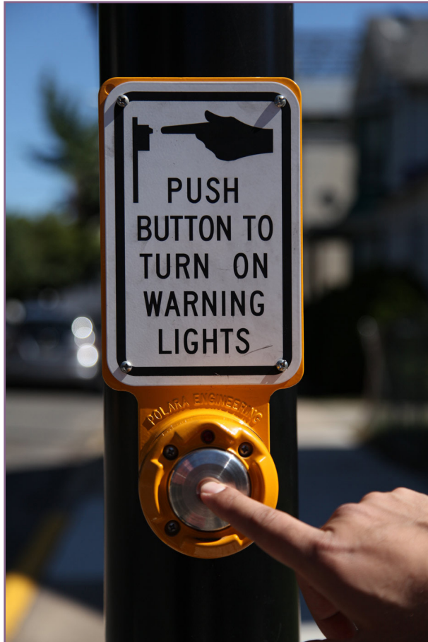
Figure 24. Refuge islands can include features such as pedestrian push buttons, MUTCD-approved signage, and beacons. ( NJDOT Bicycle and Pedestrian Resource Center )
